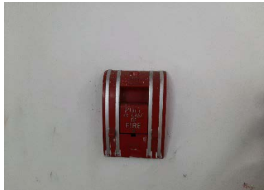
fire alarm manual station
